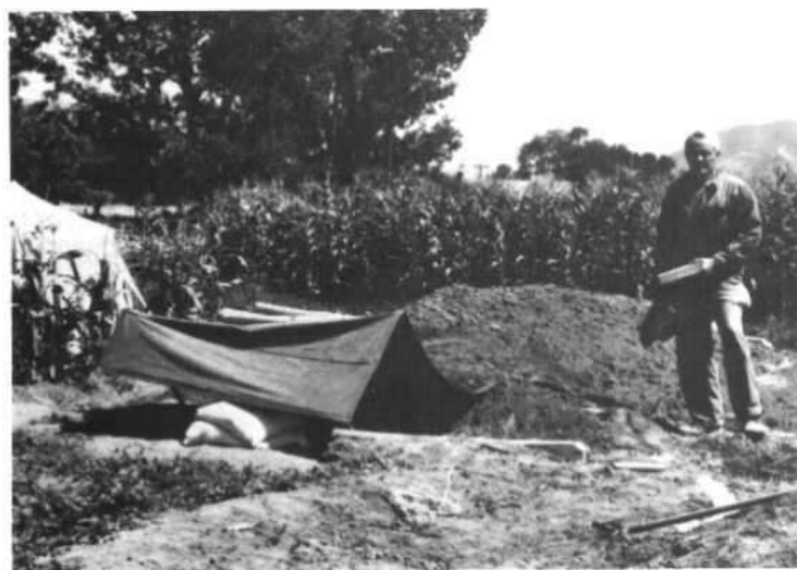
Fig. 5.6. Earth mounded over a 3 foot-wide Pole-Covered Trench Shelter. The canvas canopy would protect the vertical entry against both fallout and rain. (A smaller canopy over the air duct-emergency exit at the other end is obscured by the mounded earth.)
