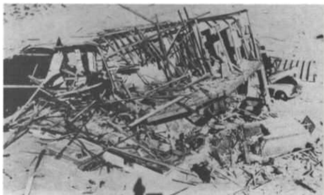
Fig. 7.4. Unburned wreckage of the same two-story, wood-frame house pictured in Fig. 7.1 after being wrecked by the 5-psi blast effects of a small nuclear test explosion.
