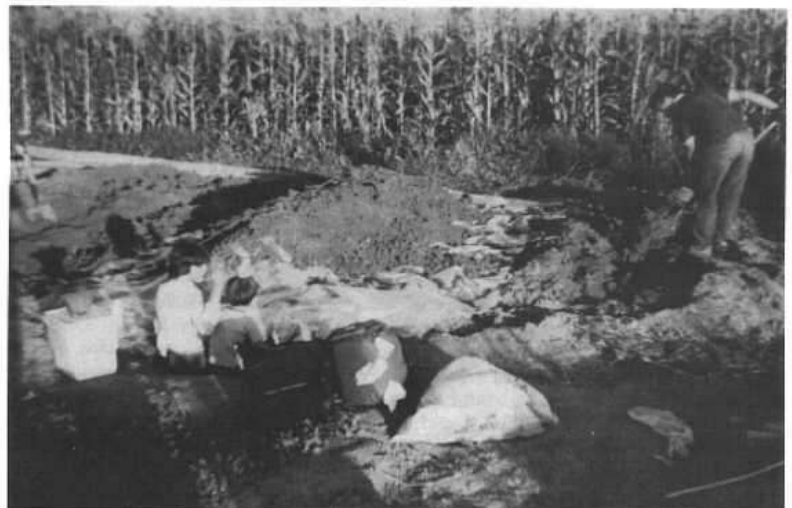
Fig. 5.4. Increasing the barrier shielding over a Pole-Covered Trench Shelter.
