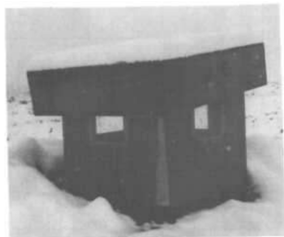
Fig. F.1, Multi-Use Emergency Exit Housing Installed Over the Square Emergency Exit Described by Figs. 17.1, 17.2, and 17.3. (Photograph)
