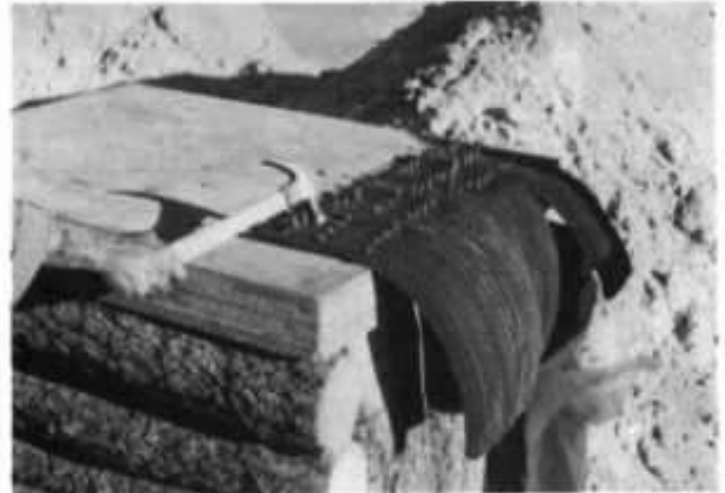
Fig. D.15. Tire-strip hinges nailed to an expedient, 4-inch-thick blast door made of plywood, designed to withstand 50-psi blast effects of very large weapons and undamaged by blast at the 53-psi range.
